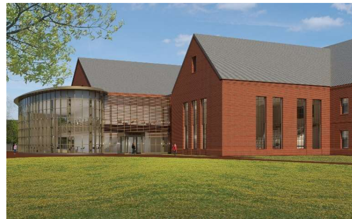
St. Mary's College Academic Building and Auditorium LEED Silver GWWO Architects with Graham Gund and Holder Construction Company (left)
