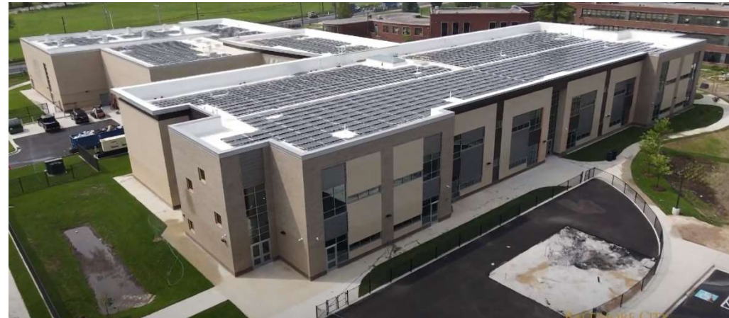
Graceland Park Elementary/Middle School Baltimore City's First Net Zero, LEED Platinum School PV Solar, Geothermal, Green Roof Grimm and Parker Architects CAM Construction (Construction Completed September 2020) Achieved LEED Platinum in 2021
