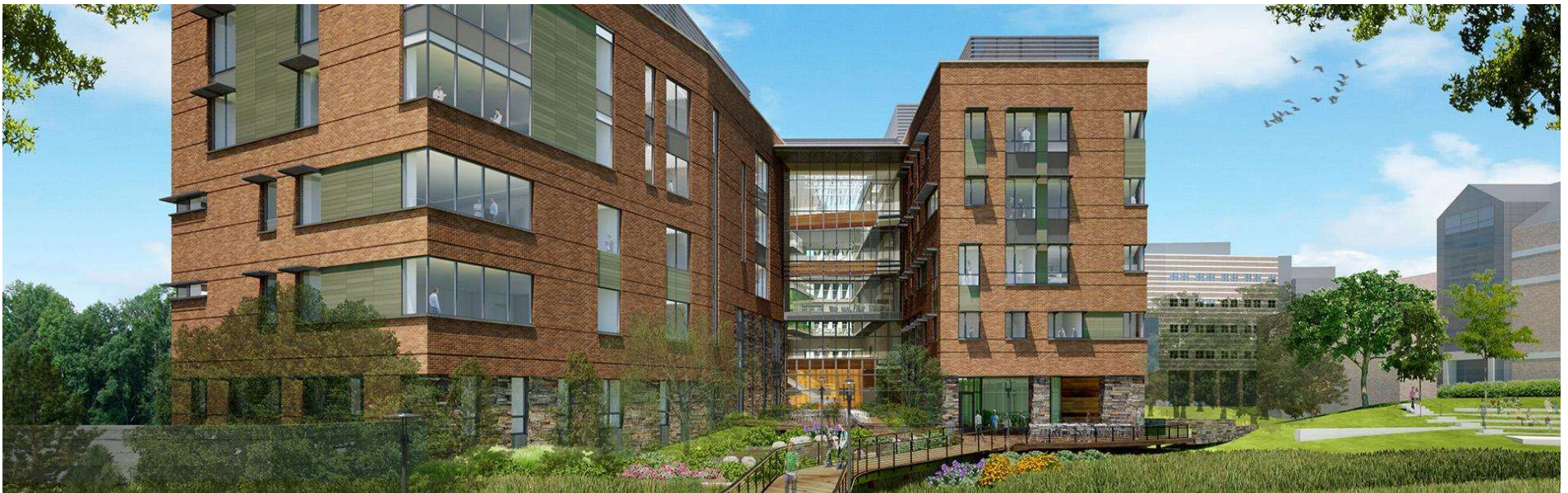
University System of Maryland at Shady Grove Biomedical Science and Engineering Educational Facility - LEED Platinum Certified June 2021
